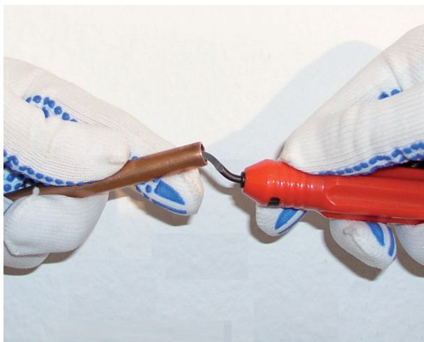
Figura 54 - Removendo as rebarbas
